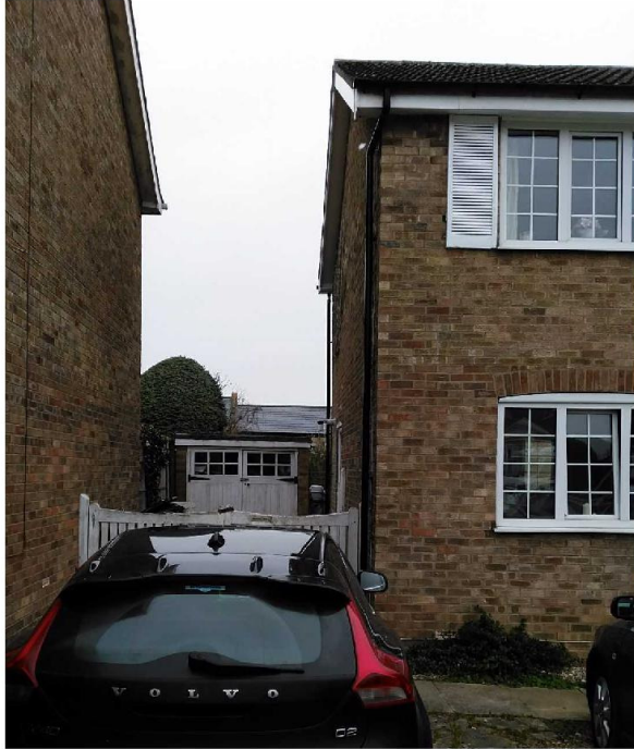
Photograph 2. View of the set back garage to be demolished
